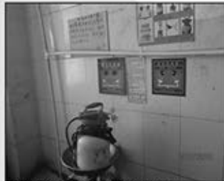
Photo of the inside of the main production hall Eye washing equipment.JPG
